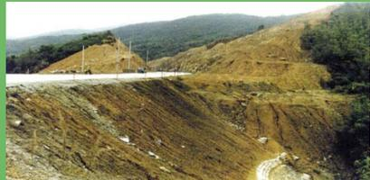
China - unstable highway fill prior to VS treatment. Road stability was so bad in untreated state that major lateral cracks in the pavement occurred
